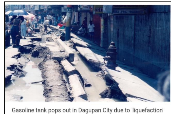
Source: Gasoline tank pops out in Dagupan City due to 'liquefaction' (Online Image) n.d. Retrieved May 30, 2020 from https://www.phivolcs.dost.gov.ph/index.php/earthquake/earthquake-hazards
